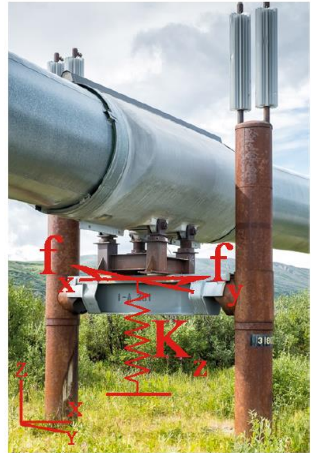
Figure: Case study of Trans-Alaska pipeline system support condition 1
